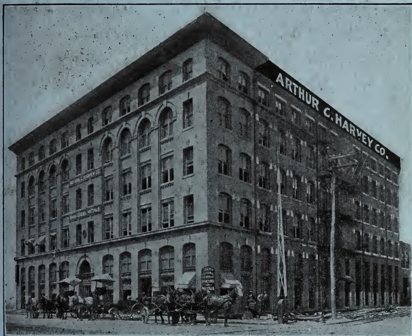
VIEW OF WAREHOUSE FROM SOUTHEAST
